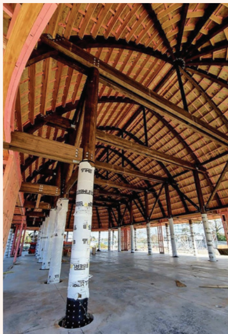
K'aute Pasifika fale construction in progress
